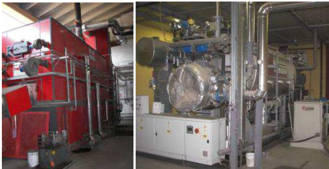
Figure 65. Thermal oil boiler rated 2 MW(th) and combined with a ORC 200 kWe turbo generator installed in a pelletizing plant in Italy. The plant is fed with class B1 woodchips; its consumption is approx. 7,000 t/year.
