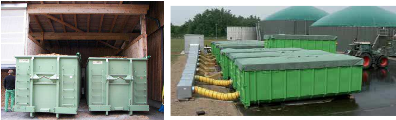
Figure 47. On the left, a dryer-container supply with by-heat from a small CHP based on wood gasification. On the right the same solution applied to a CHP-biogas plant.
