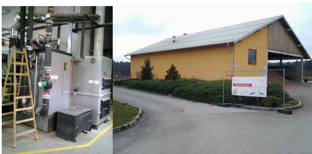
Figure 40. 1.3 MW woodchip boiler plant, Revital Kidričevo.
