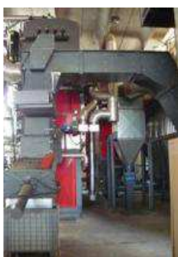
Figure 66. ORC plant (185 kWe) with micro turbine combined with a saturated steam boiler (20 bar, 2.5 MWth).
