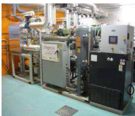
Figure 66. ORC plant (185 kWe) with micro turbine combined with a saturated steam boiler (20 bar, 2.5 MWth).
