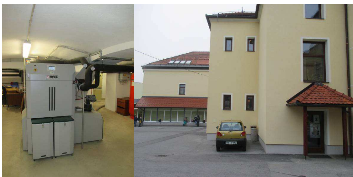
Figure 41. Wood pellet 200 kW boiler at the Cirkulane Primary School.
