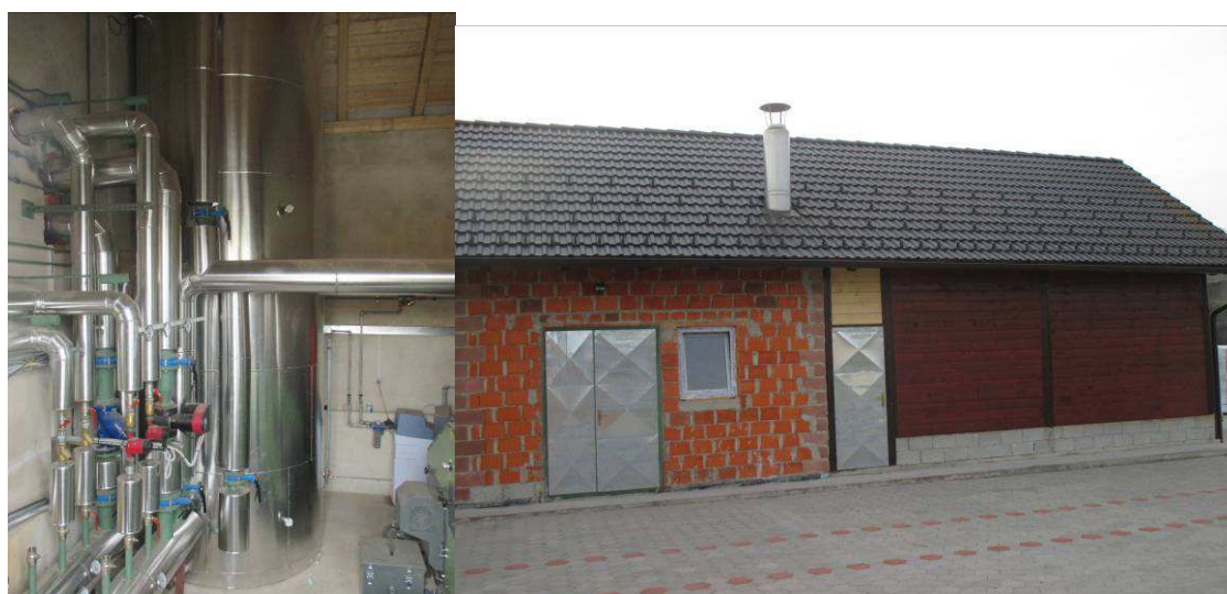
Figure 39. Greenhouse heating woodchip boiler plant.
