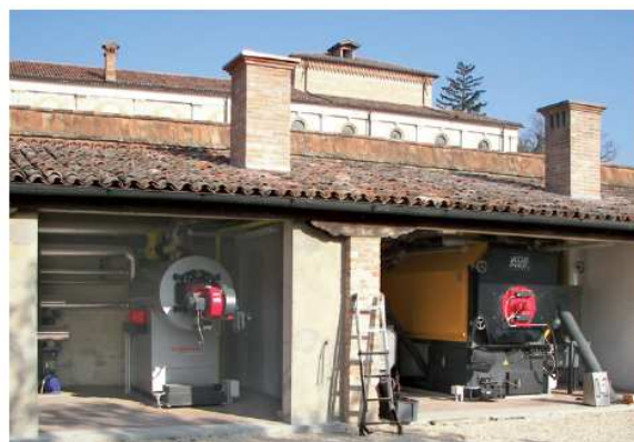
Figure 63. Annual heat load curve using the woodchips–natural gas combination, peak and minimum loads. On the right a plant equipped with a woodchip boiler 540 kW is provided.
