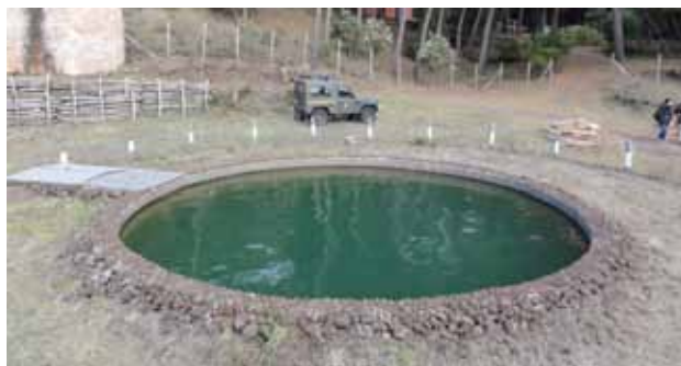
Photo 10: Fire-fighting facilities set up by the State Forestry Corps. A pool of water designed for helicopter water bombers with reservoir (top left).
