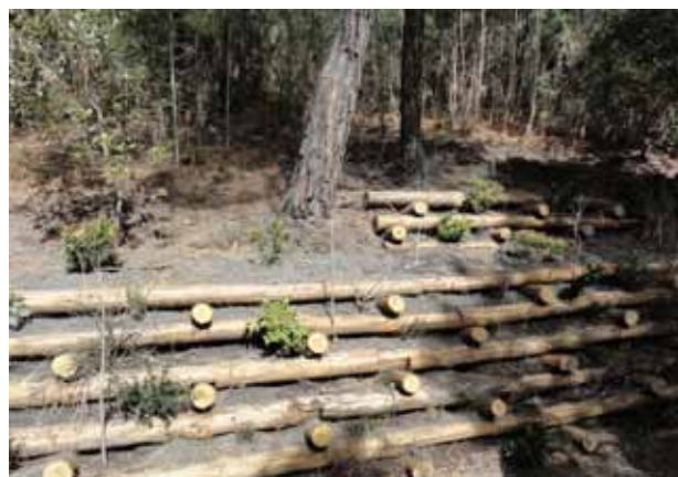
Photo 9: Experimental ecological engineering works, including along the trails in the Tirone Alto Vesuvio reserve, allow the development of a diversified vegetation type to permanently retain soil.
