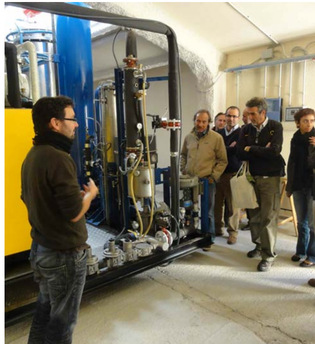
Photo 11: Micro-generation unit (biomass gasification and electric power generation).
