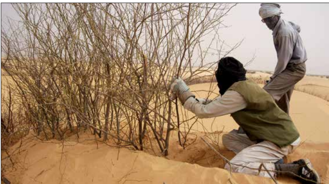
Installing a palisade, mechanical dune stabilization, Mauritania
